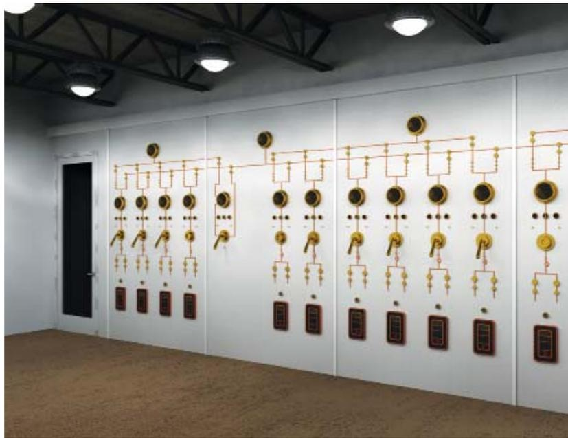
**Adequate lighting for vertical surfaces, such as control panels, is important for keeping daily operations running smoothly – and critical in emergencies. Follow your lighting system's maintenance requirements, which will depend on light source and location.** Photos: Holophane
